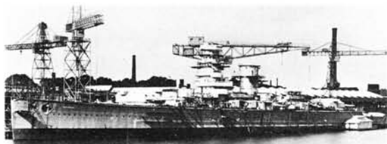
The Graf Spee in the fitting-out basin. Now the medium guns are already in position and funnel and tower-mast are erected.
